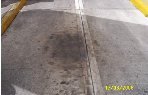
Figure 1. The stained concrete pavement before MicroCat-SMPL application
