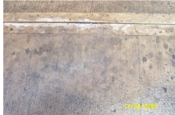
Figure 2. The stained area after MicroCat-SMPL application
