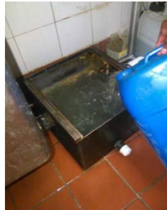
Cleaning/Disinfection of Trap
